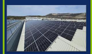
Photovoltaic panels => 40% of electricity demand
