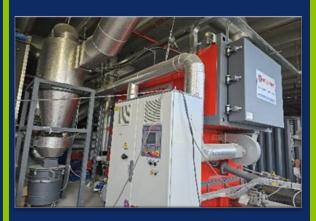
1 MW **biomass boiler** operating on wood pellets
